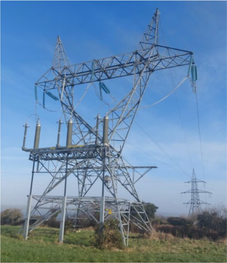
Figure 3.10: Line Cable Interface Mast
