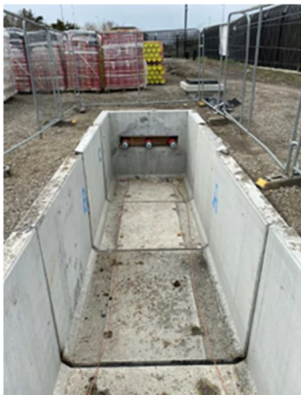
Figure 3.8: Pre-cast Joint Bay prior to Cable Installation
