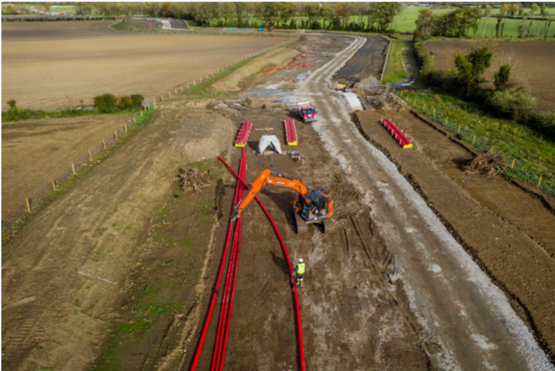
Figure 3.6: Typical underground cable construction in agricultural lands
