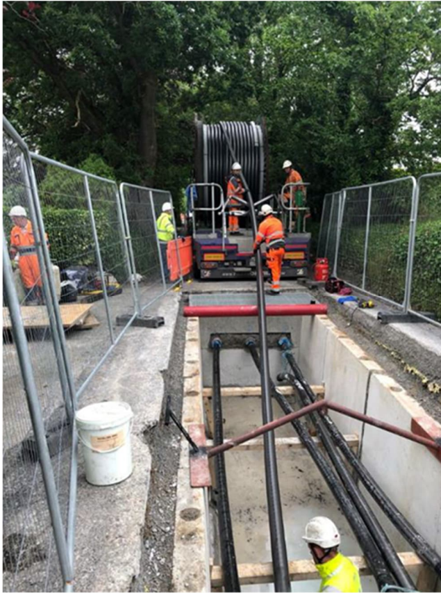
Figure 3.9: Typical Set-Up of HV Cable Pulling Procedure
